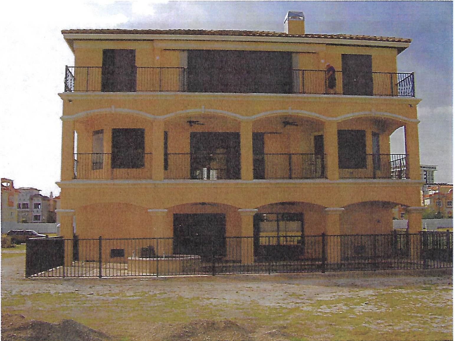
REAR VIEW PICTURE TAKEN ON 3-12-08
