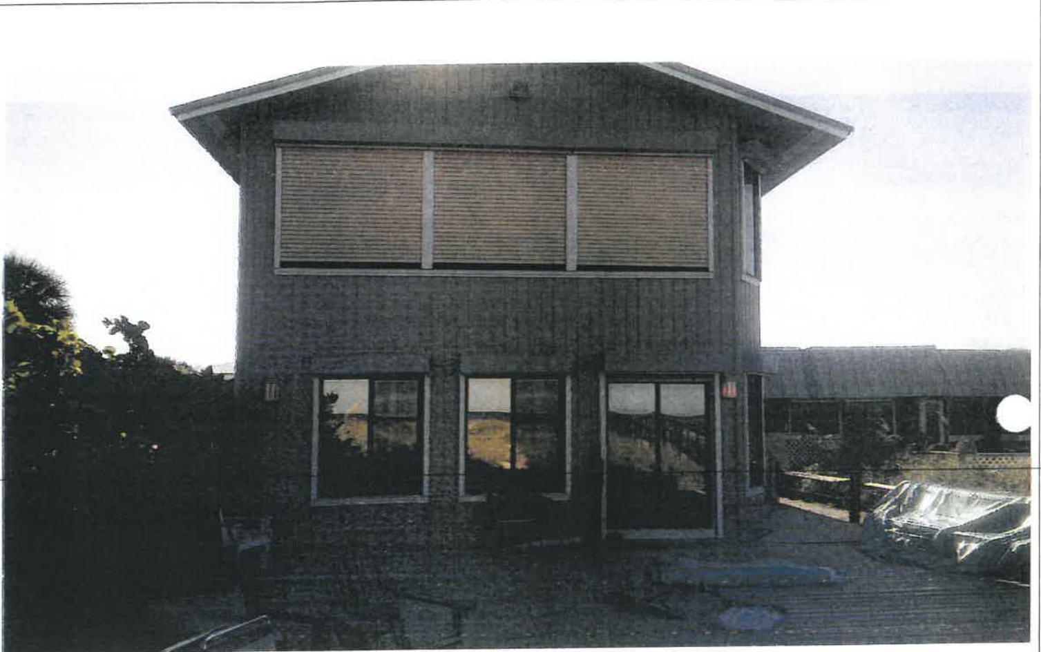
REAR VIEW Picture taken on: 8-17-2015
