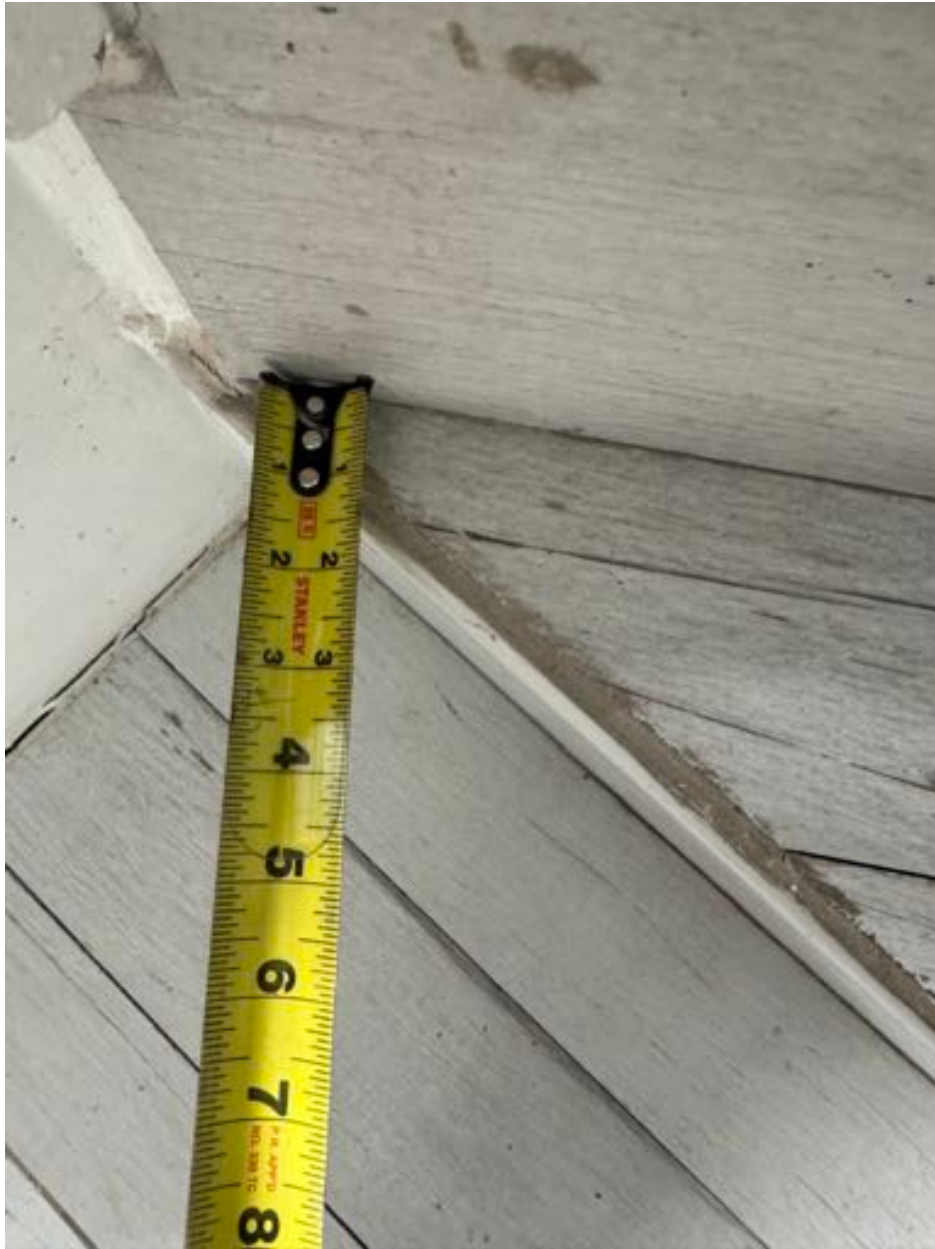
(Minimum width of winder step is not to code, and comes to a point. The first photo demonstrates where 6" would be if it were to code.)
